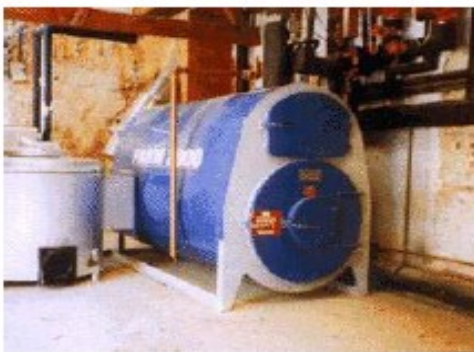
Figure 4. Farm 2000. Suitable for heating farm buildings and estates; will burn a variety of fuels
